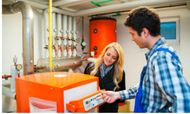
Figure17 A German engineer introduces the performance of energy-saving equipment Source: Research report titled Providing Economic Incentives and Promoting Energy Efficiency Improvement
