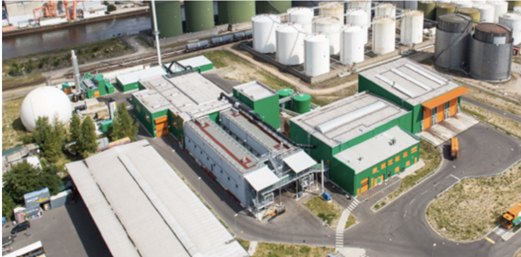
Figure 7: View of the waste digestion facility with biogas upgrading plant in the upper-left corner (Source: BSR)
