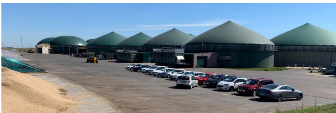
Figure 9: Birds-eye view of the biomethane production plant
